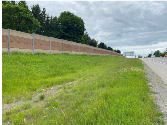
Photo 2: Engineered slope, ditching and highway, evidence of previous disturbance, facing southwest
