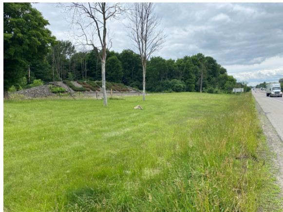
Photo 4: Graded slope and ditching abutting shoulder of highway, facing southwest
