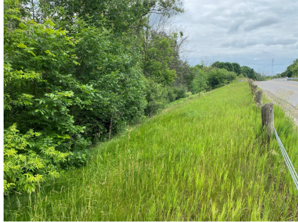
Photo 6: Engineered slope of overpass leading down to forested area, facing south
